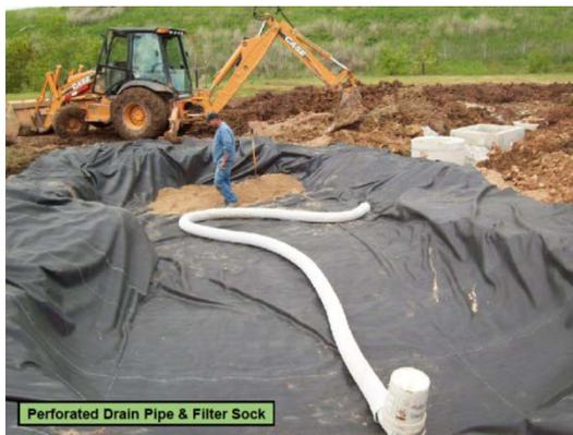
Figure4. Plastic liner used for each system.
